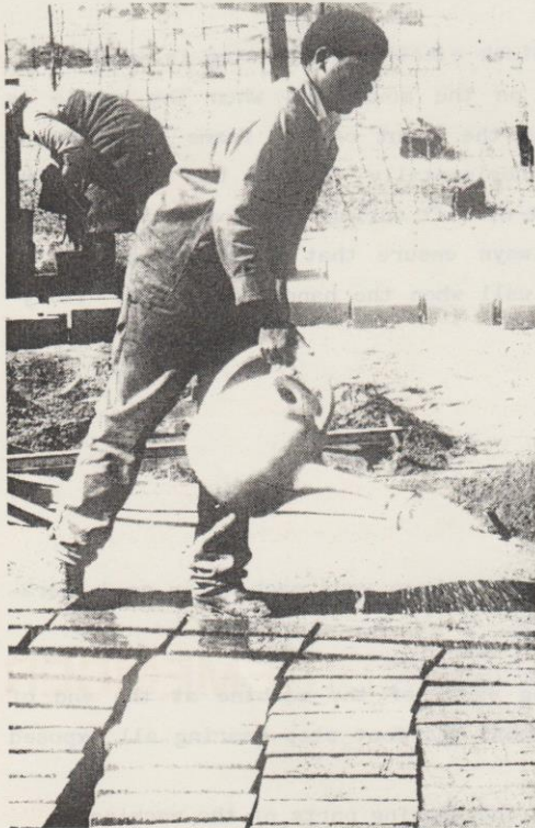
Figure 23 Watering the Bricks
